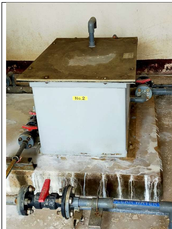
Photo 3: Constant head tanks for feeding bleaching powder solution
