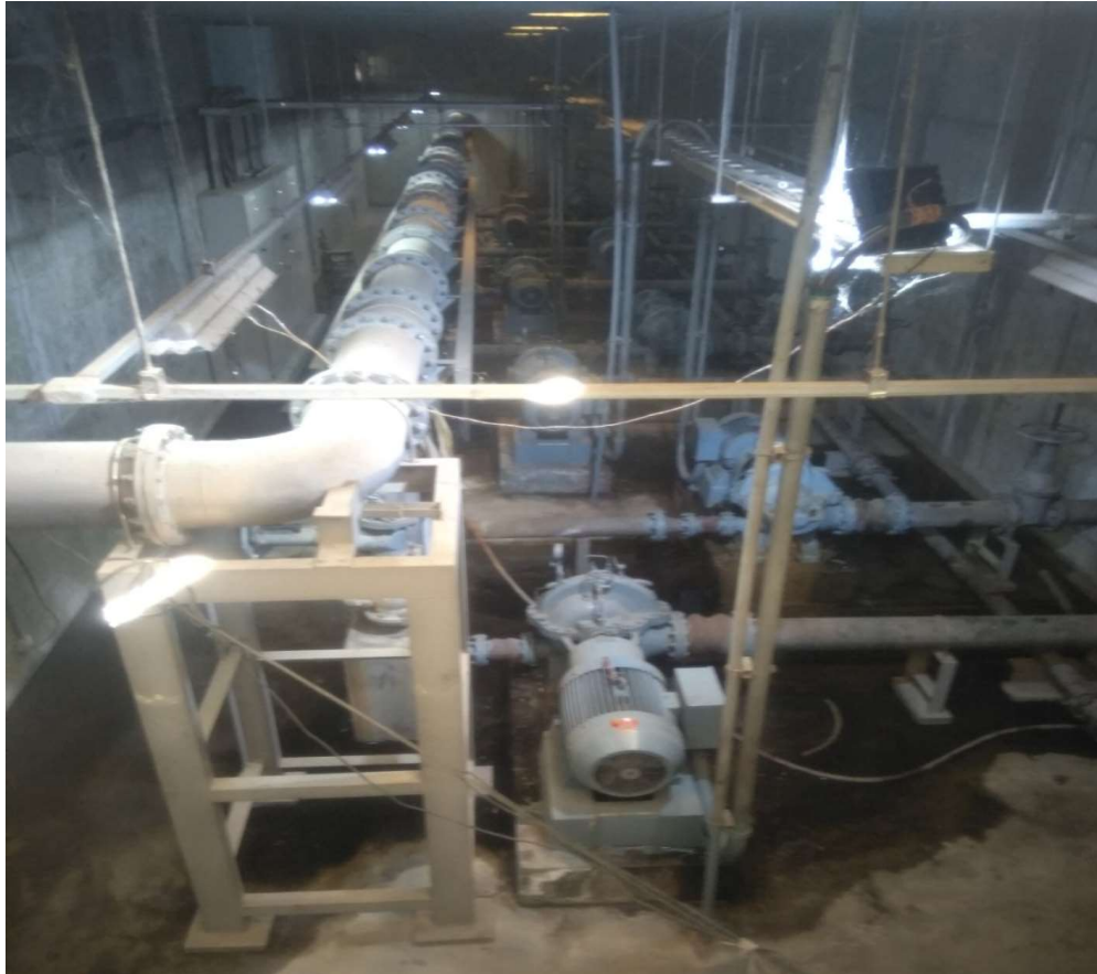
Figure 18: Transmission pumps
