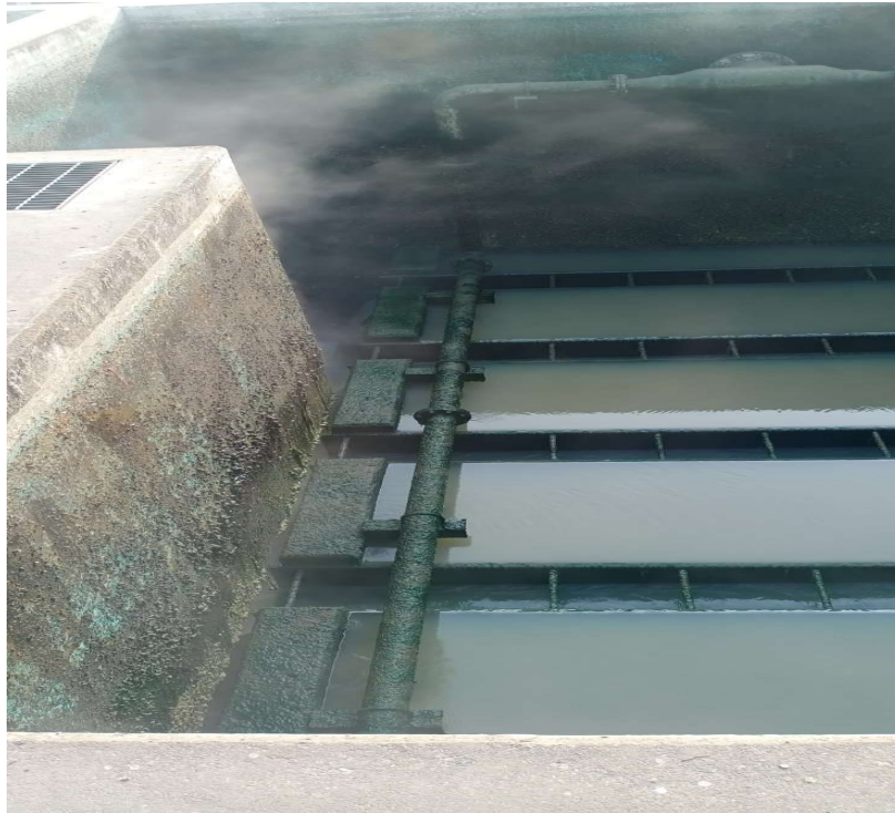
Figure 16: Rapid sand filter
