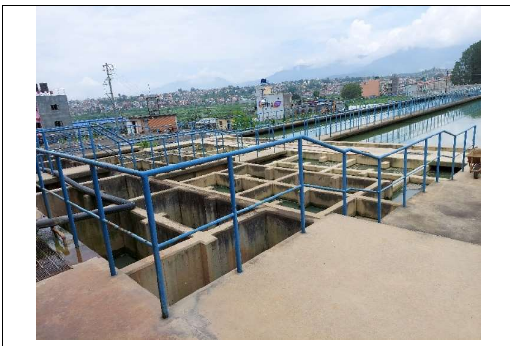
Figure 2: Flocculation basin
