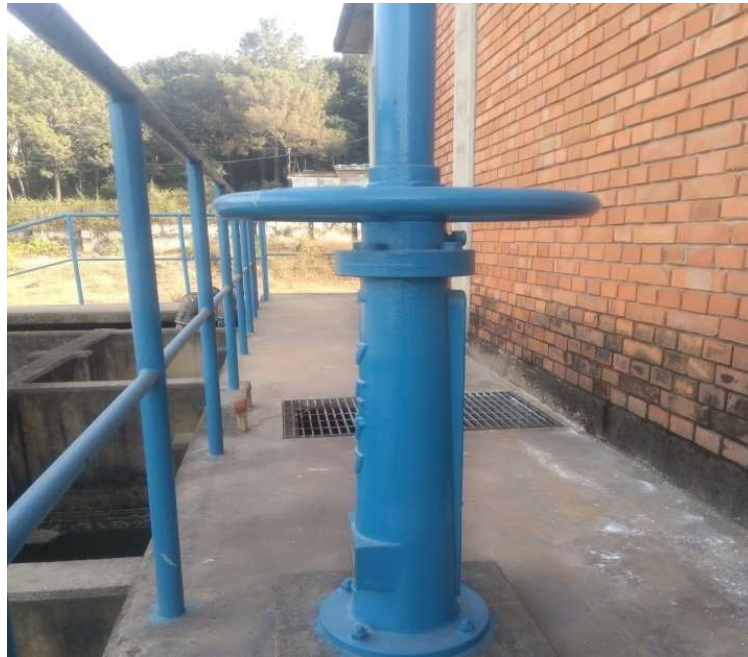
Figure 26:Raw Water Inflow Gate
