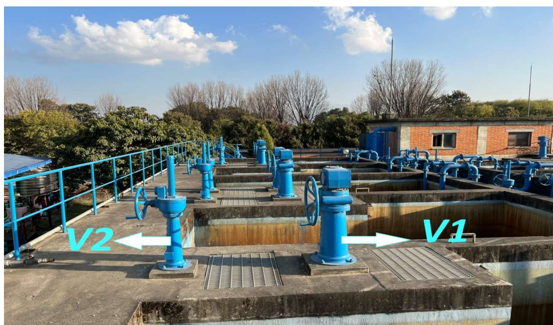
Figure 3: Water inflow and drainage valves
