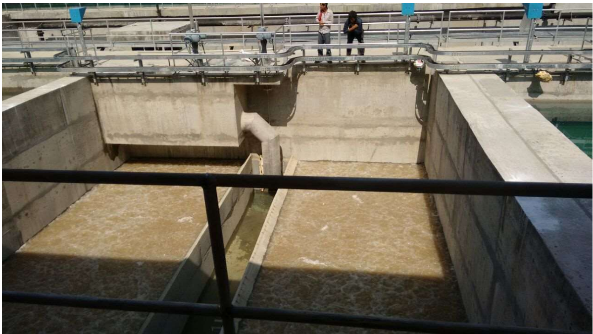
Photo 13: Backwashing in progress
