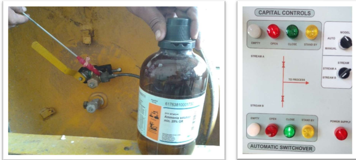
Photo 30: Automatic Stream selection panel
