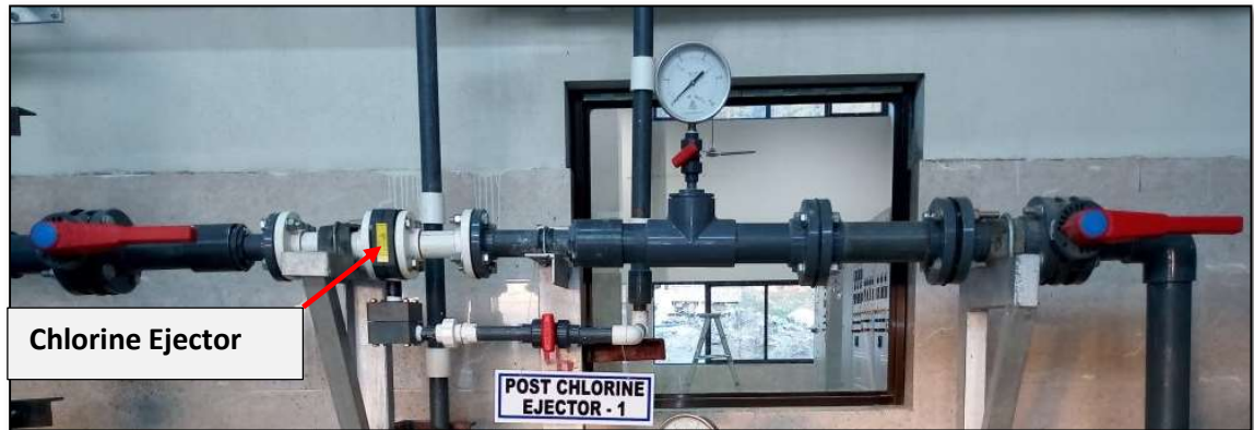
Photo 28: Chlorine Ejectors
