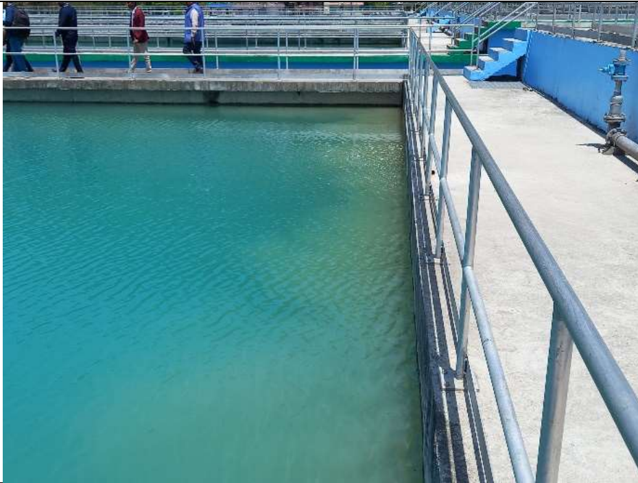
Inlet of Sedimentation Basin
