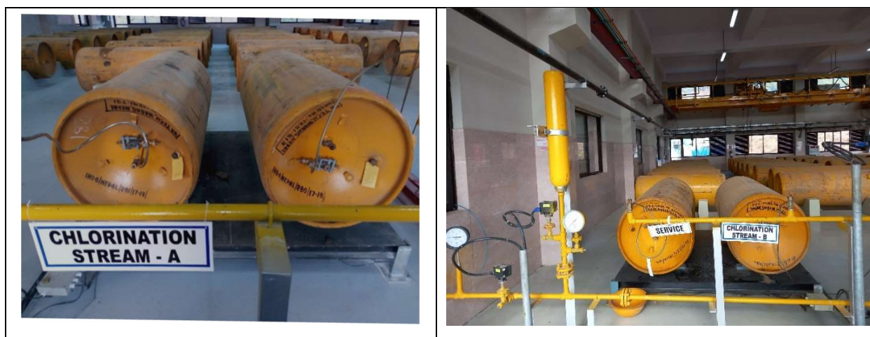
Photo 25: Chlorine cylinders
