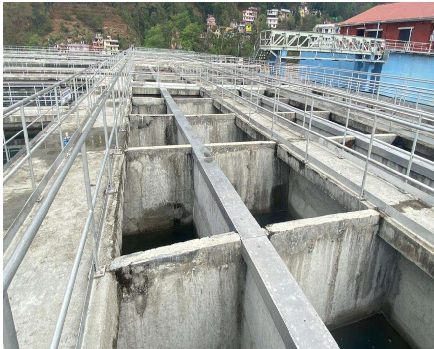
Photo 5: Flocculation Basins
