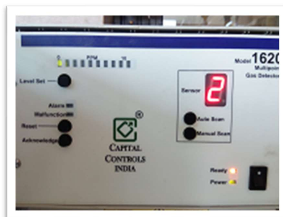
Figure 18: Chlorine Gas leak detector Control unit
